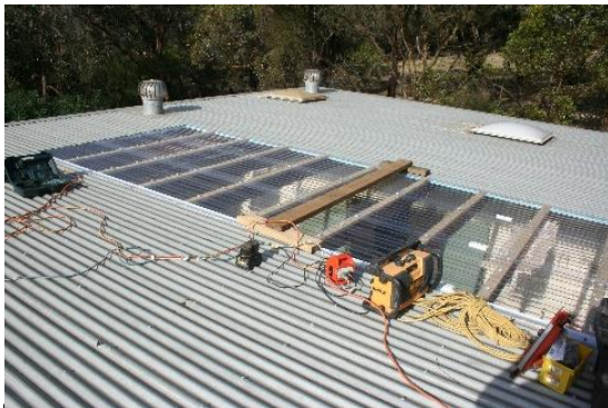
Polycarbonate installation in shed roof
